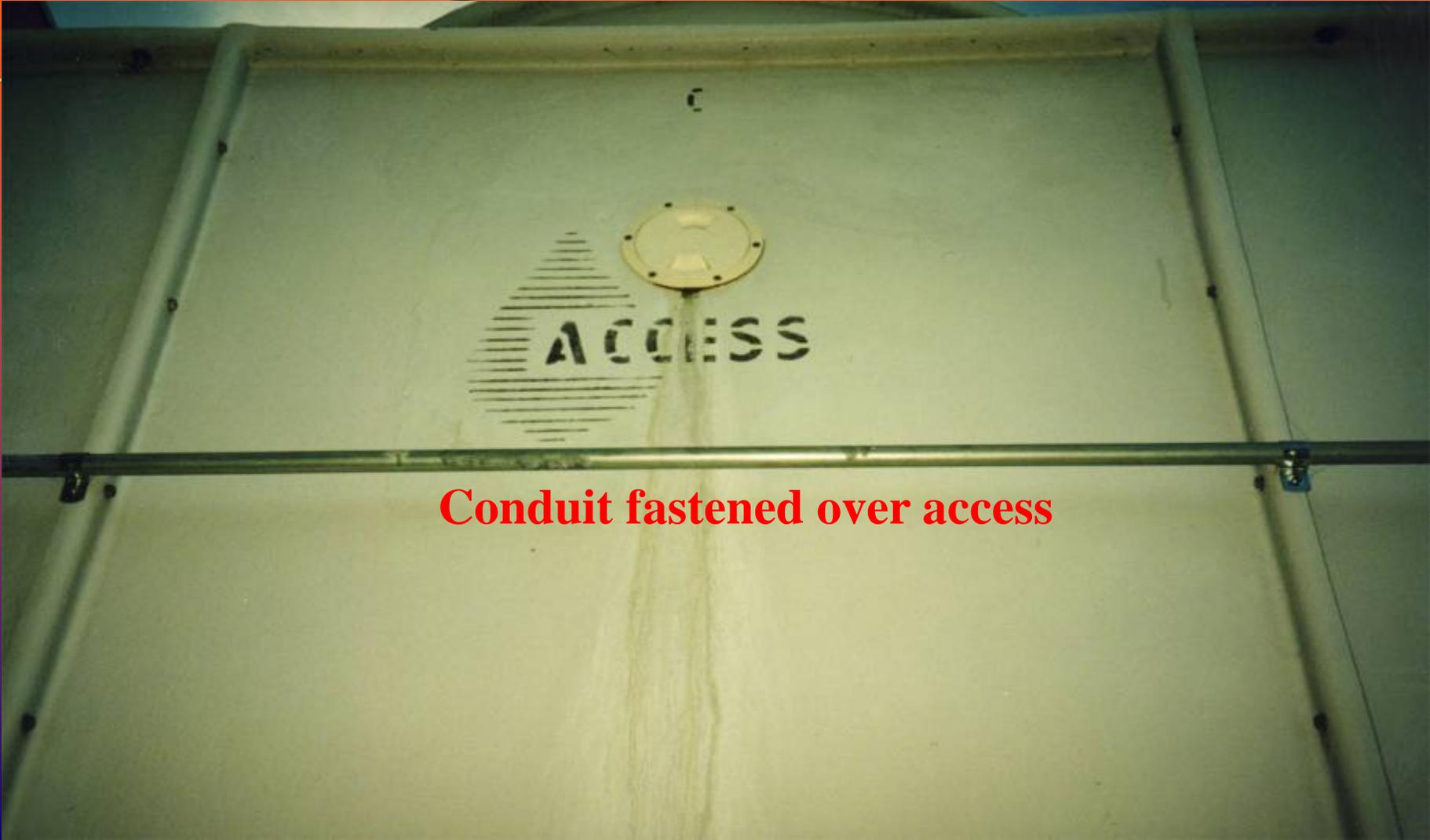
**Conduit fastened over access**
