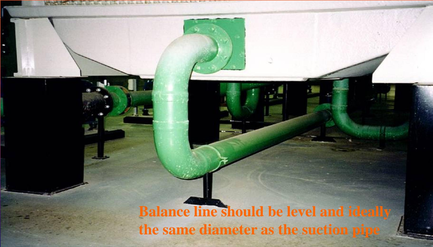
**Balance line should be level and ideally the same diameter as the suction pipe**
