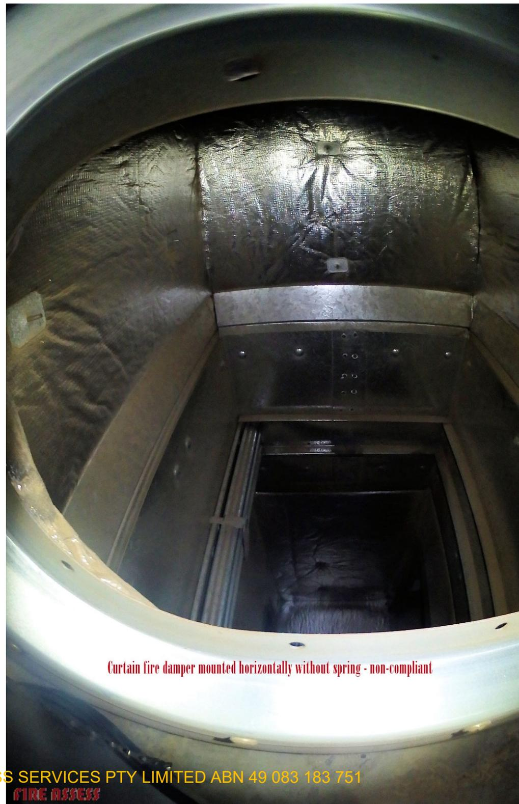
*Curtain fire damper mounted horizontally without spring - non-compliant*
