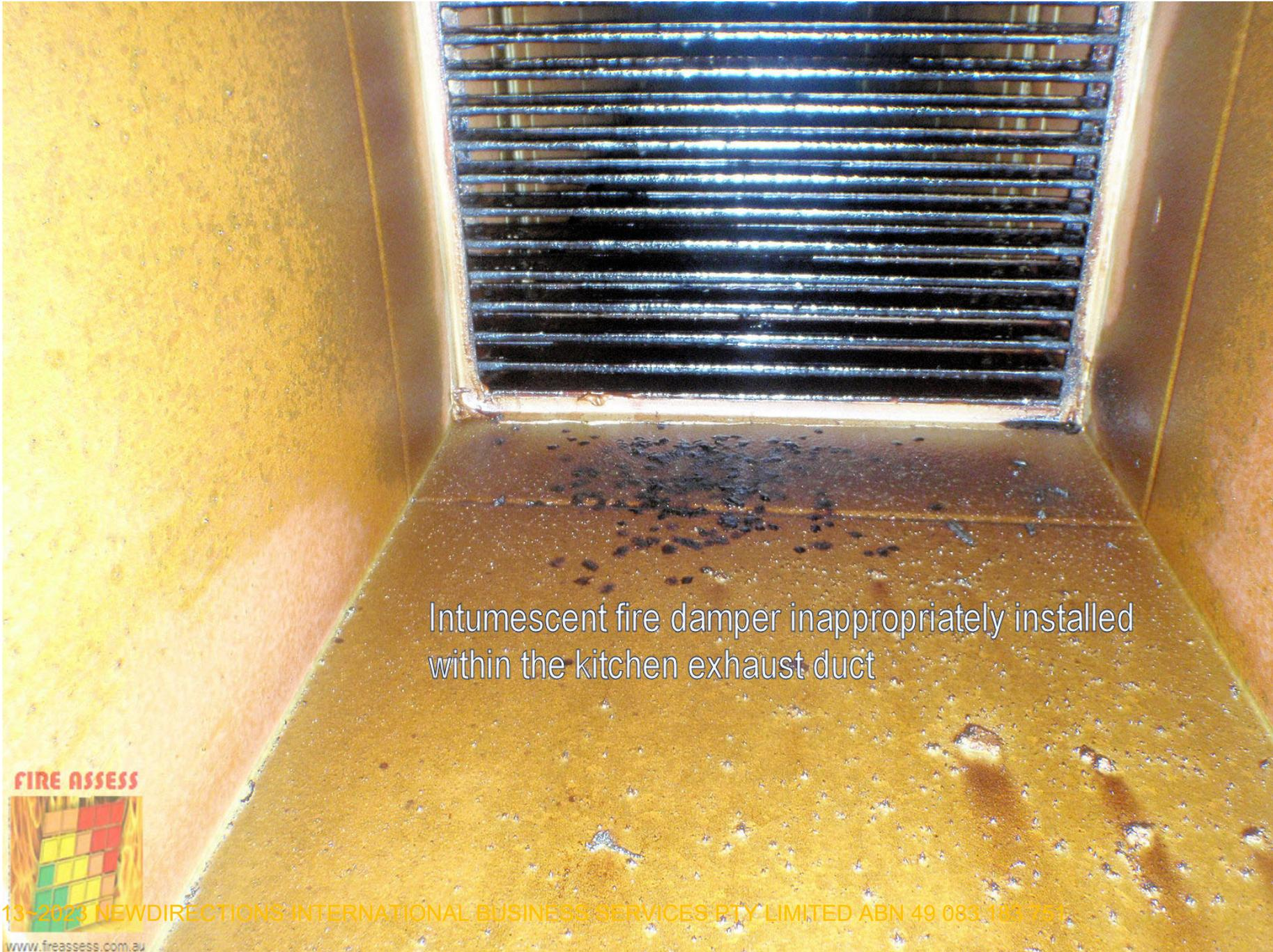
Intumescent fire damper inappropriately installed within the kitchen exhaust duct
